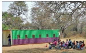
Kindergarten in the shade while finishing touches are put on the new container school
